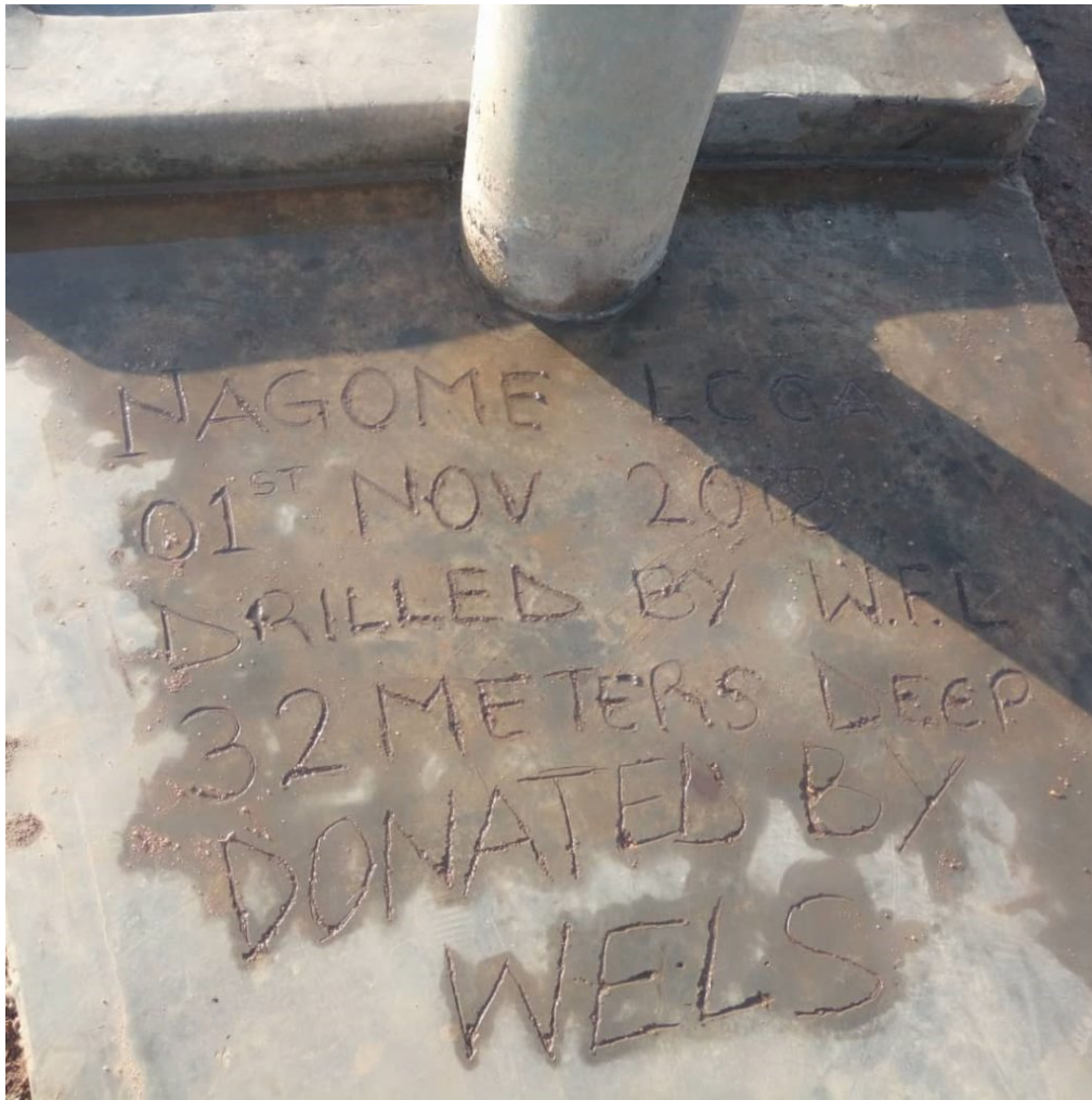
The cement base for water run-off on the Nagome well
