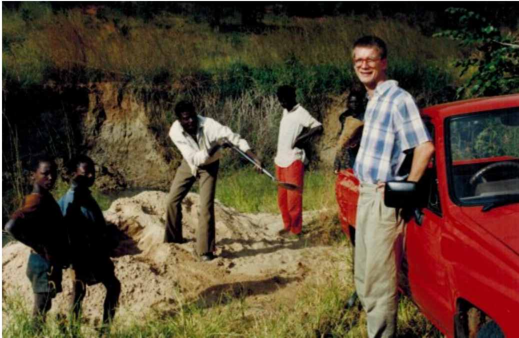
Hauling sand for church building projects in Mzuzu - 1995
