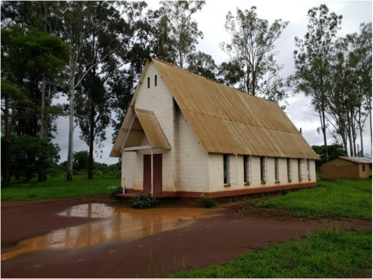
This is the first church (though refurbished) that was built by the mission in Mwembezhi.
